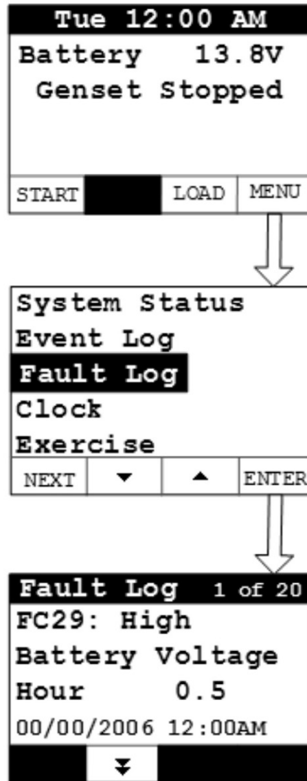
FIGURE 15. FAULT LOG SCREEN
