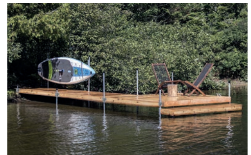
Make small stationary dock sections to ease winter removal.
