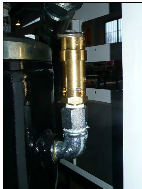
Figure 12.1-1 Control of the safety valve
