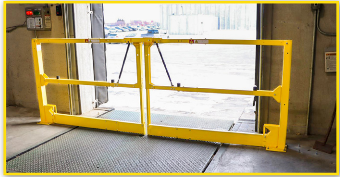
Loading Dock Preparation/Fall Protection
