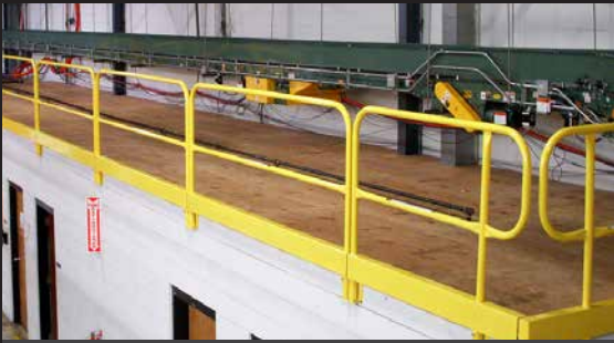
MECHANICAL SERVICE AREAS
