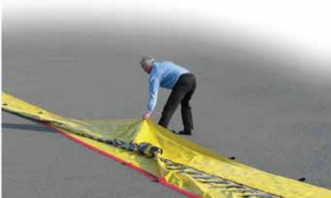
1 - Completely unfold the Water-Gate.
