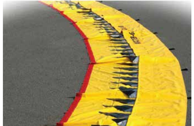
2 - Curve the Water-Gate as needed, making sure the back of the Water-Gate is not stretched.
