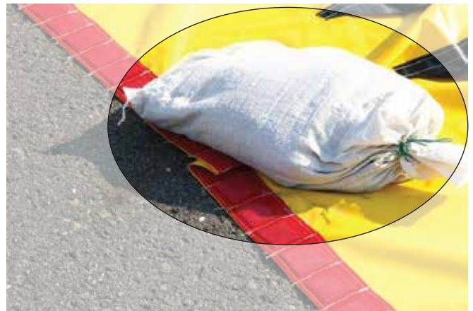
4 - Sandbags can also be used to close off the spaces or folds formed by the Water-Gate ballast weights.
