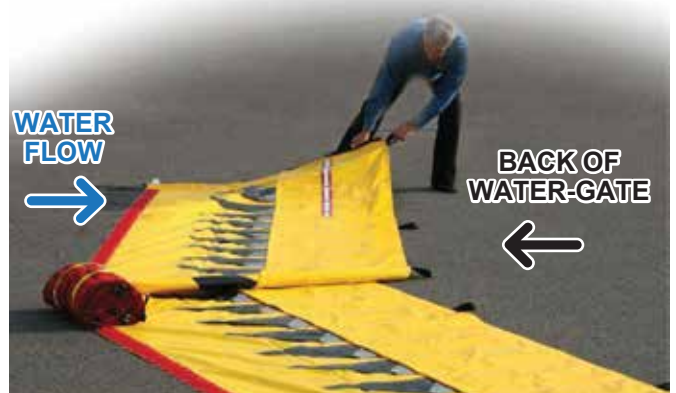
2 - Place ballast weights on the front flap of the Water-Gate and turn to the desired angle.
