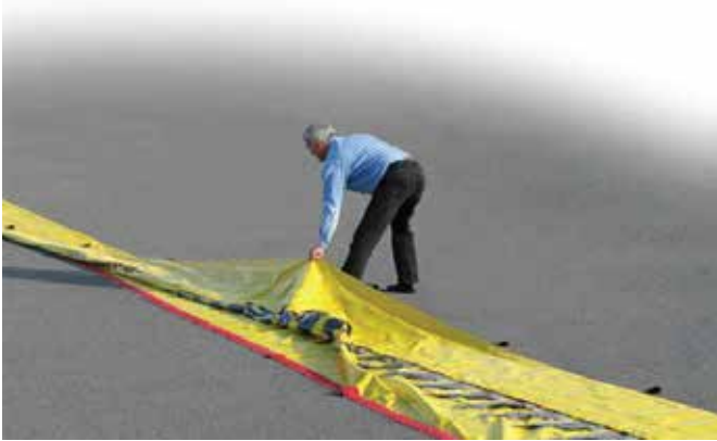
1 - Completely unfold the Water-Gate.
