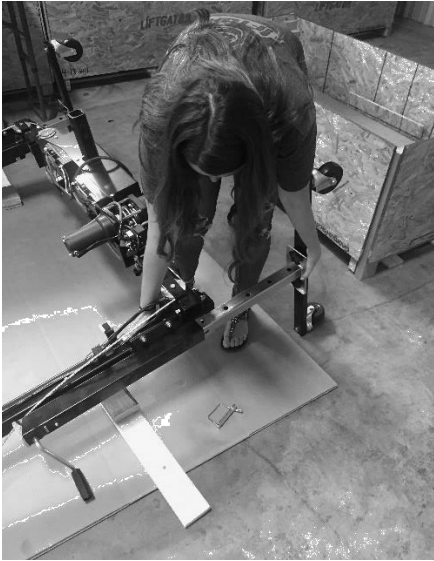
16. Lift the frame assembly and insert the support legs into the adjuster body.
