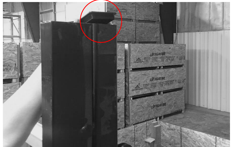
57. Install caps on top of upright rails.
