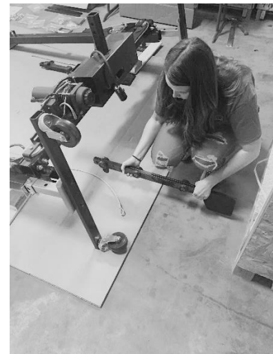
27. Route the wire rope under the crossmember and toward the bottom of the upright rails.
