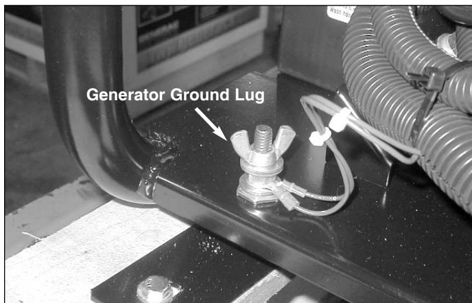
Figure 13 - Grounding the Generator
