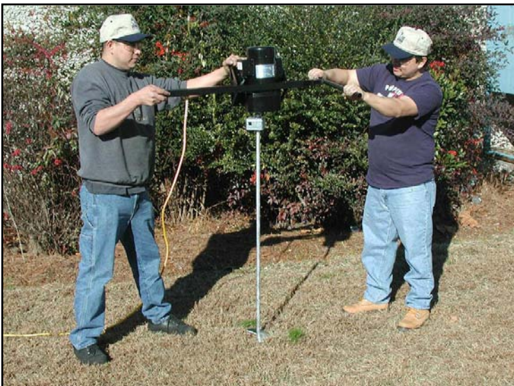
Two man operation makes easy work of anchor installation
