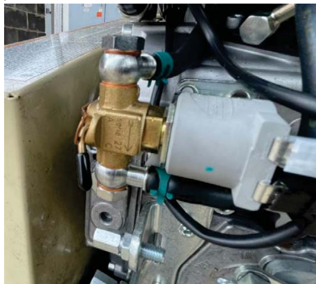
Kohler diesel engine fuel solenoid valve (Shown in transport position)
